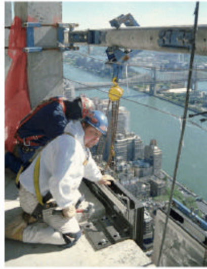
Figure 10: Panel Suspended from Trolley Ready for Final Installation
